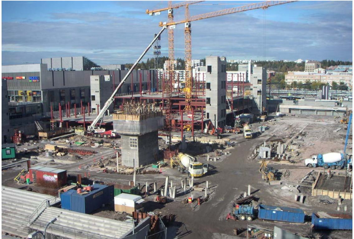
Figure 6. Construction site for the shopping center Sello in Leppävaara, Espoo. (Photograph: Finnmap Consulting Oy, 2004)
